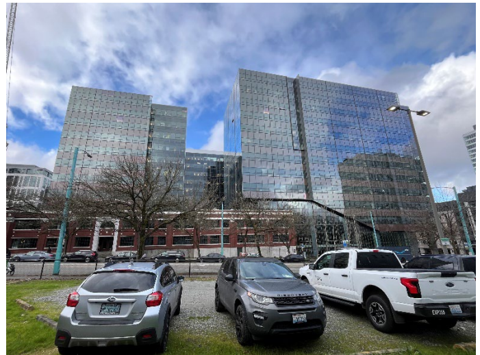
Troy Laundry cleanup site, 2026
