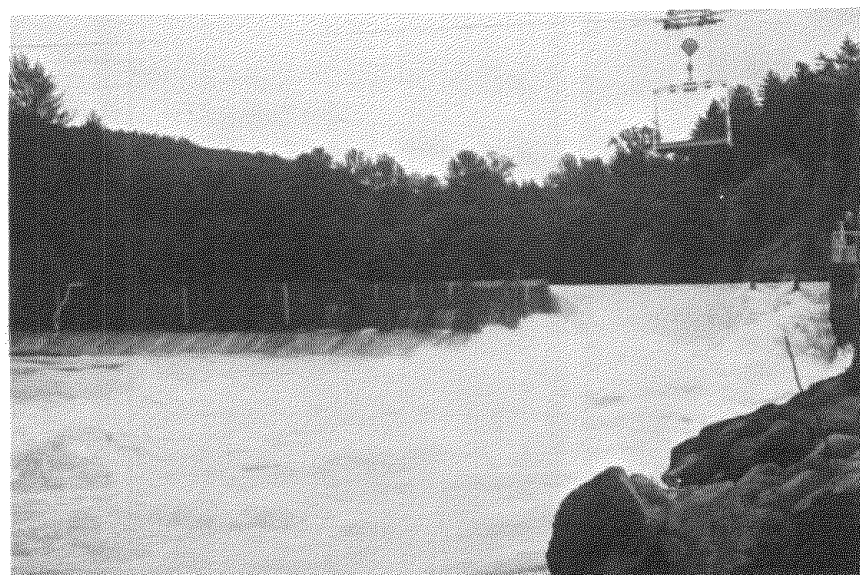
PUGET SOUND POWER & LIGHT CO. DIVERSION DAM - Showing Discharge with Flume Gates Closed and 7-6 Ft. Wide Sections of Dam Removed 7/29-76
