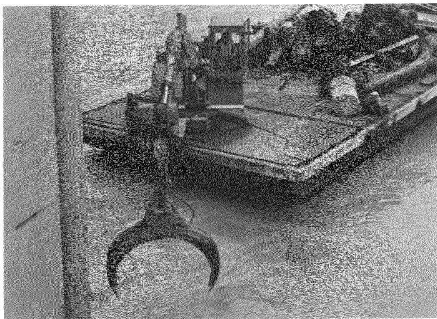
Work Barge - Showing Debris Tongs 8/12/76
