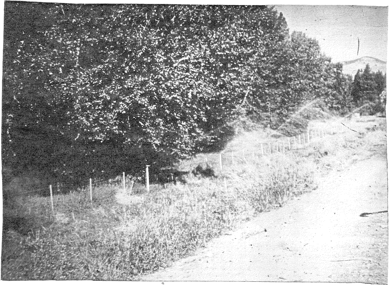
Appendix A, Figure 2. Spray-irrigation line #2 adjacent to the Methow River (looking west), Winthrop WTP, 8/84.
