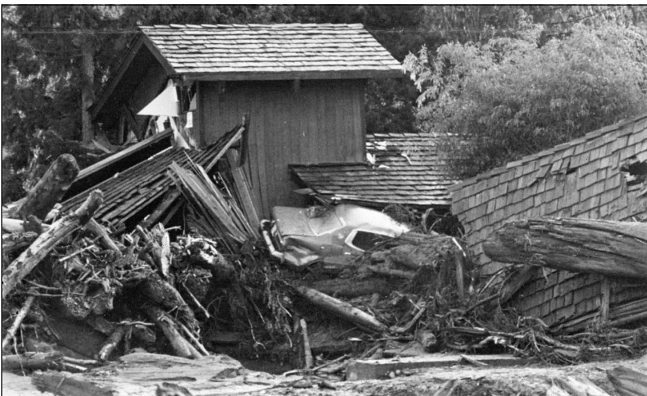
Flood hazard areas are prone to mud slides and debris flow damage. (Whatcom County, 1983)
