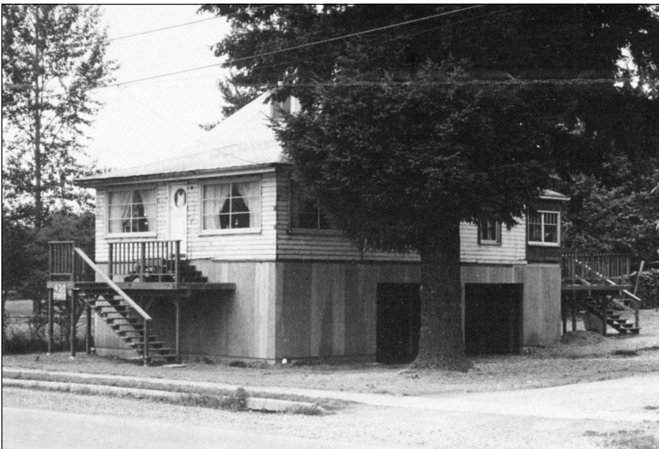
If you live in a flood hazard area, you should consider elevating your house. (Skagit County)
