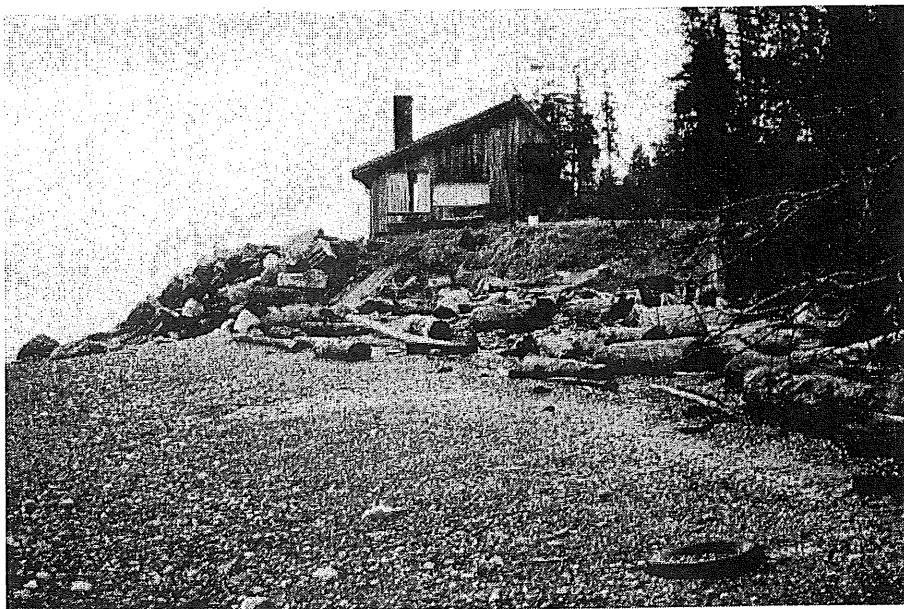
Figure 10. Cabin constructed on artificial promontory seen in Figure 9. (Photo: 1997)
