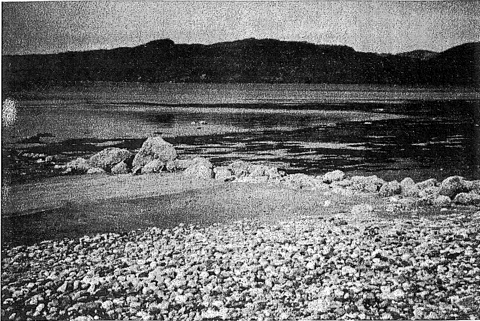
Figure 11. Largest of groins seen in Figure 9. (Photo: 1997)
