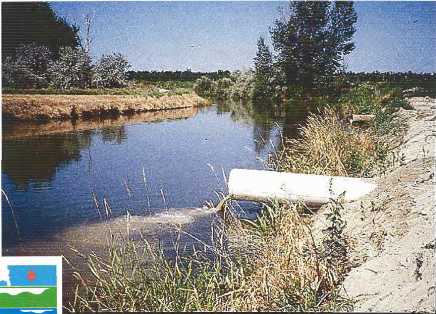
RETURN DRAIN TO THE SUNNYSIDE VALLEY IRRIGATION CANAL
