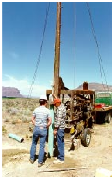
Ecology well-drilling inspector Mark Ader helps a landowner install a well correctly.
