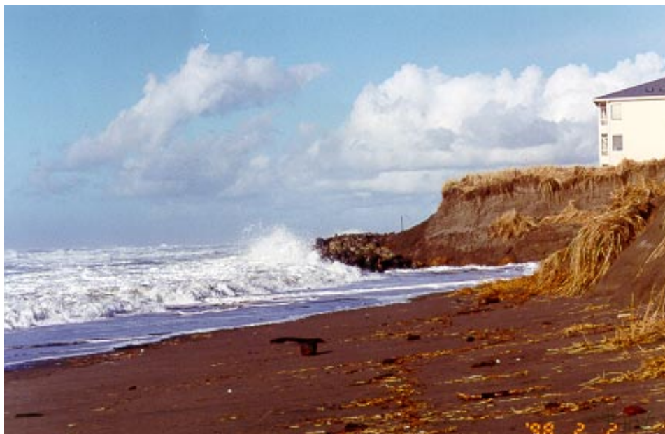
Erosion is threatening this Ocean Shores condominium. The owners built a temporary rock wall to protect the property.
