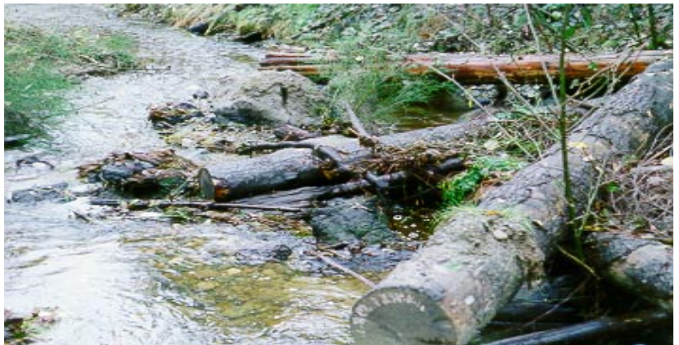
A new law (HB 2879) exempts some fishery enhancement projects, such as adding woody debris to streams, from certain regulations and permit fees. Photo: Jeff Legg
