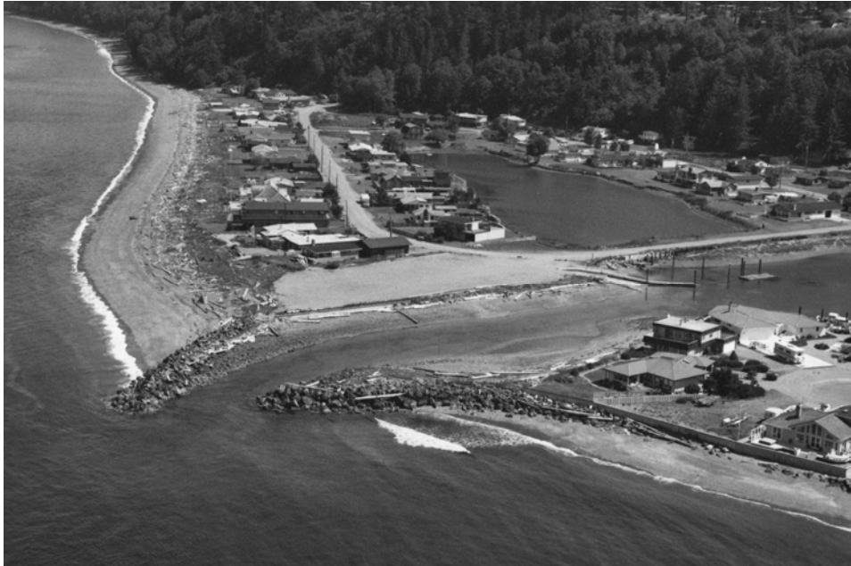
Figure 16. Erosion caused by interrupted littoral drift.
