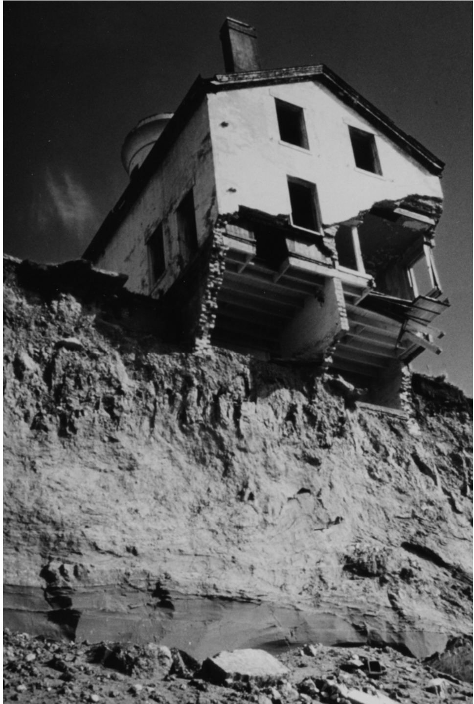
Figure 5. Smith Island lighthouse (1979 photo). The lighthouse is essentially gone today. Anticipating erosion rates (here more than 2 ft/yr) and the vulnerability of such landmarks can guide your decisions about when and where to install a reference station.
