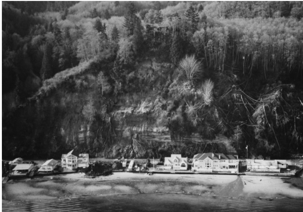
Figure 15. Waterfront homes built on fill obtained by excavation of lower bank. Bulkheads built on the beach retained the fill as it was placed. The lower bank is now nearly vertical. The removal of erosional debris from the access road along the toe of this bank has now replaced wave action as an “agent of erosion”.
