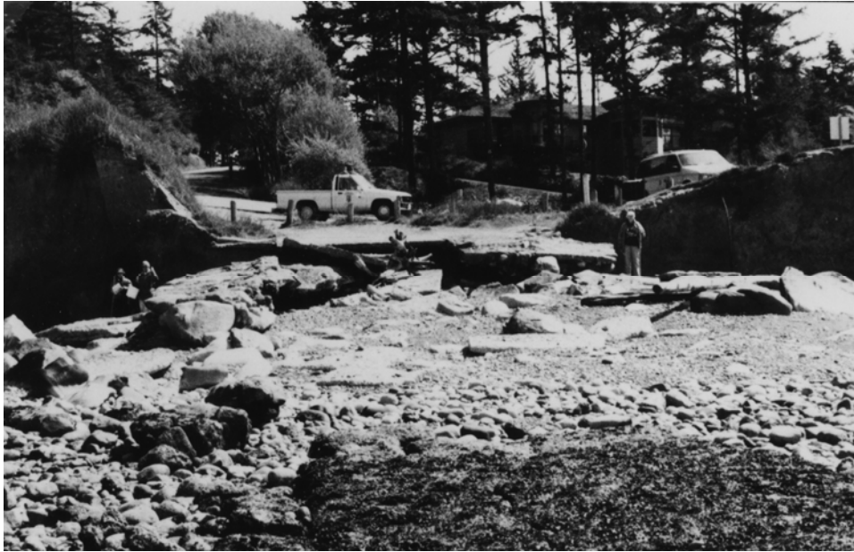
Figure 8. The now-defunct boat launch at west end of Libbey Road. The ramp has been acting as a beach groin , slowing right-to-left longshore drift. Note differences in elevation of people standing on upper beach on either side of the ramp. The bank on left has no beach to protect it and is eroding faster than on the right. What will happen when the ramp is totally destroyed?
