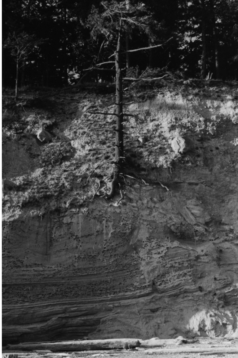
Figure 3. Accelerated erosion of bluff toe. The 100+-year-old tree at mid-bank indicates negligible erosion of the upper bank. In contrast, the lower bank here has eroded almost 30 feet. How long will it take for this accelerated erosion to reach the upper edge of the bluff?
