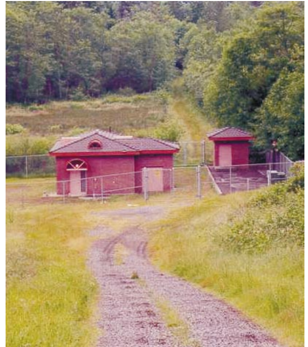
This pump station sends raw sewage from Black Diamond to the Metro treatment plant in Renton, 16 miles away. The discharge once went into a wetland above Lake Sawyer for treatment, but the "innovative" method didn't work.
