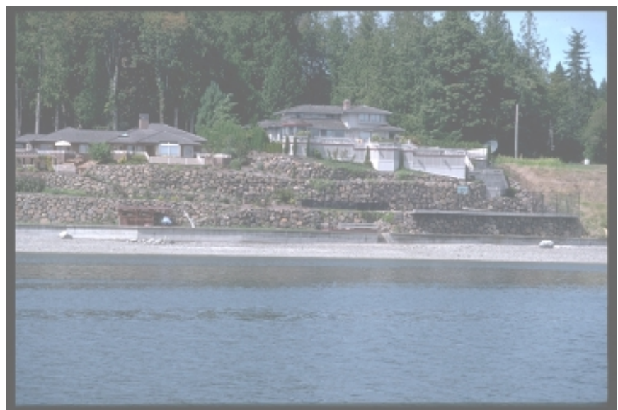
Proposed guidelines for local shoreline programs would promote environmentally-friendly methods for controlling erosion. Traditional shore defense structures, such as bulkheads (pictured), often degrade fish habitat. Photo: Hugh Shipman
