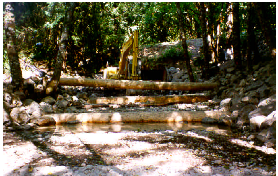
The Legislature approved up to $120 million for salmon recovery projects. Photo by John Hanson: Crews work to eliminate a salmon barrier on Little Salmon Creek.
