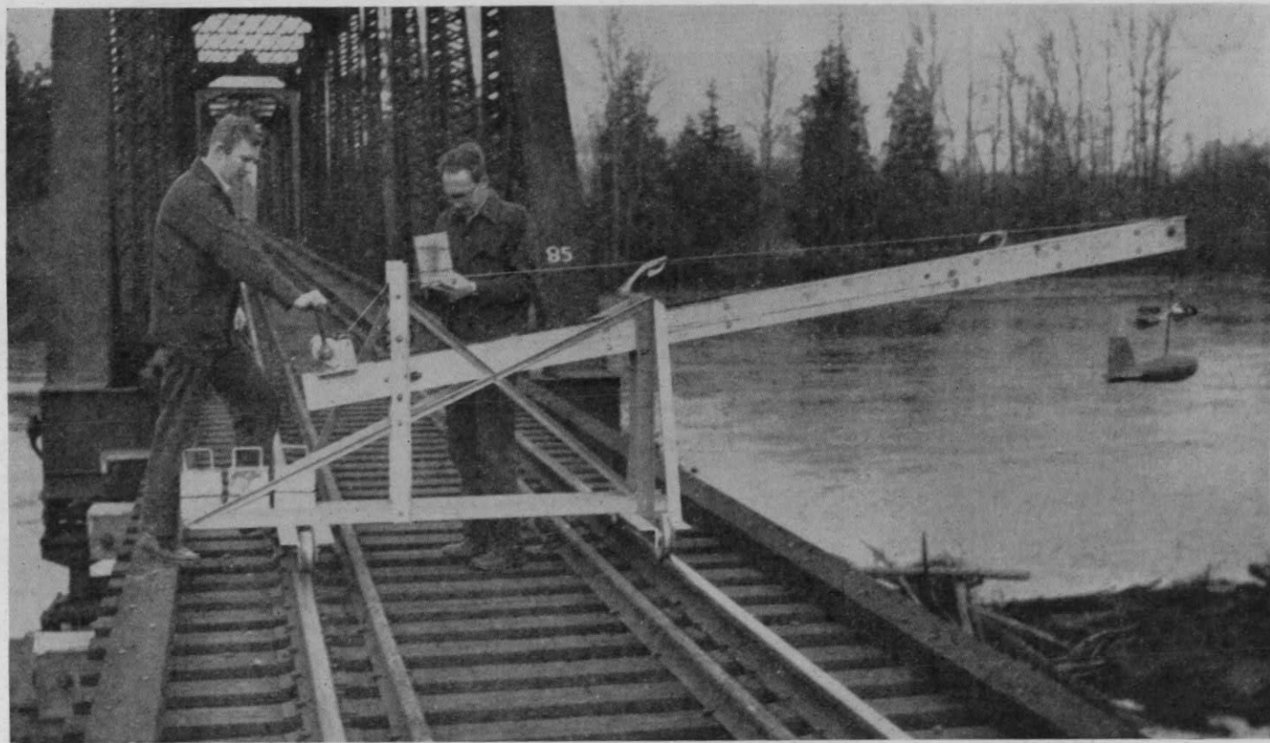
Figure 11. Discharge measurement from railway bridge. Skagit River near Sedro Woolley.
