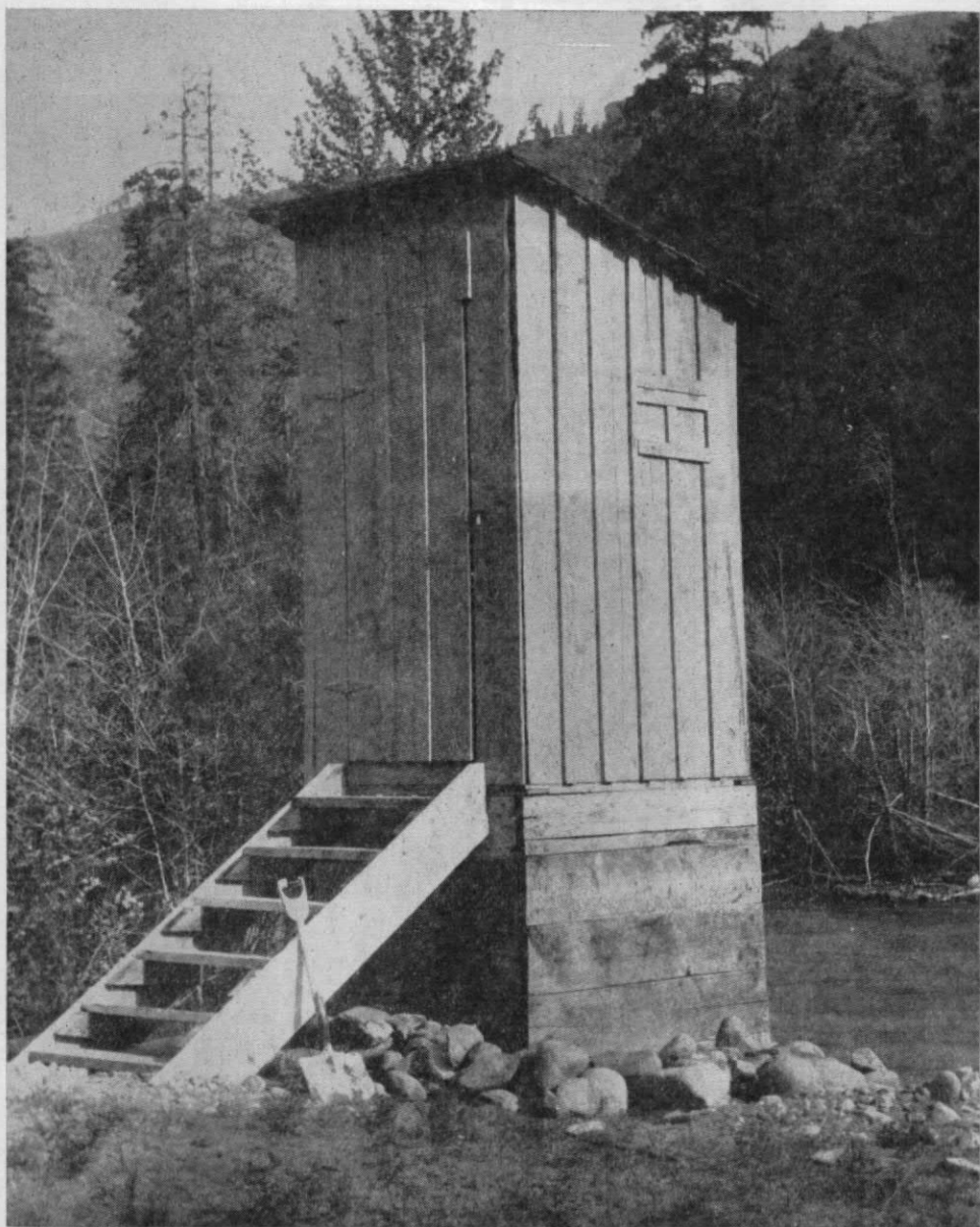
Figure 22. Early type wooden gage house and well on Tieton River at headworks of Tieton Canal, near Naches.
