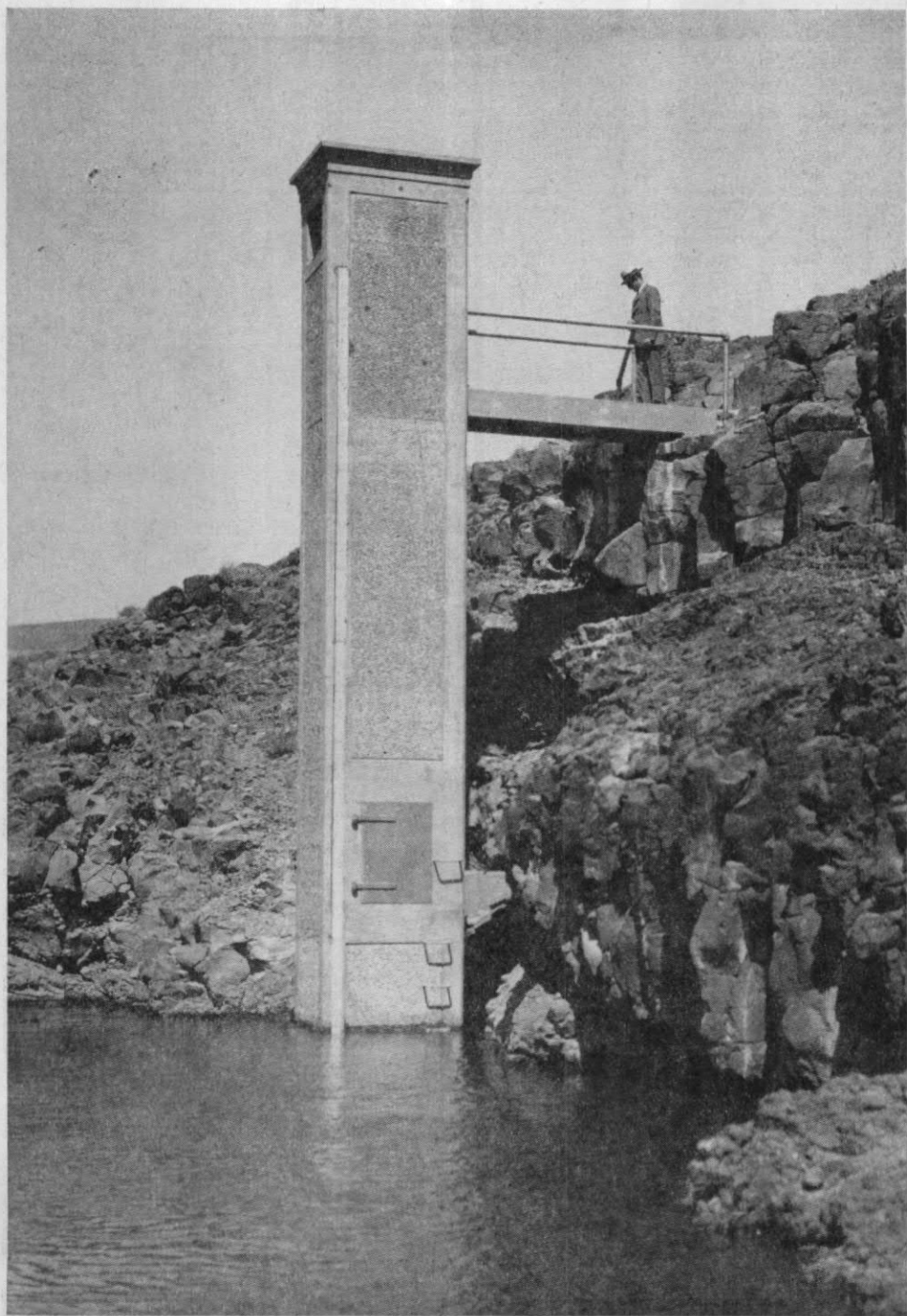
Figure 20. Concrete gage house and well on Columbia River at Trinidad.
