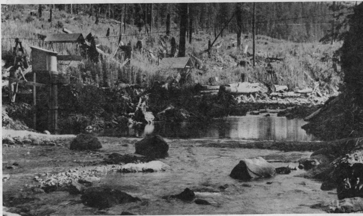
Figure 24. Gaging station in isolated area, Smay Creek near Lester. Note shelter cabin, also artificial control below gage,
