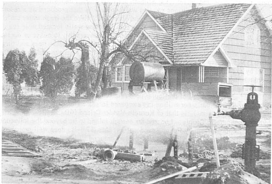
Figure 5. The J. W. Wilson well (same as Figure 4 above), showing nozzled flow after the well was capped and valved.
