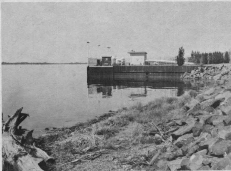
A. Pumping station at 5/27-15D. The pumps have capacities of 1500-9000 gal/min and the entire system has a capacity of about 120,000 gal/min.
