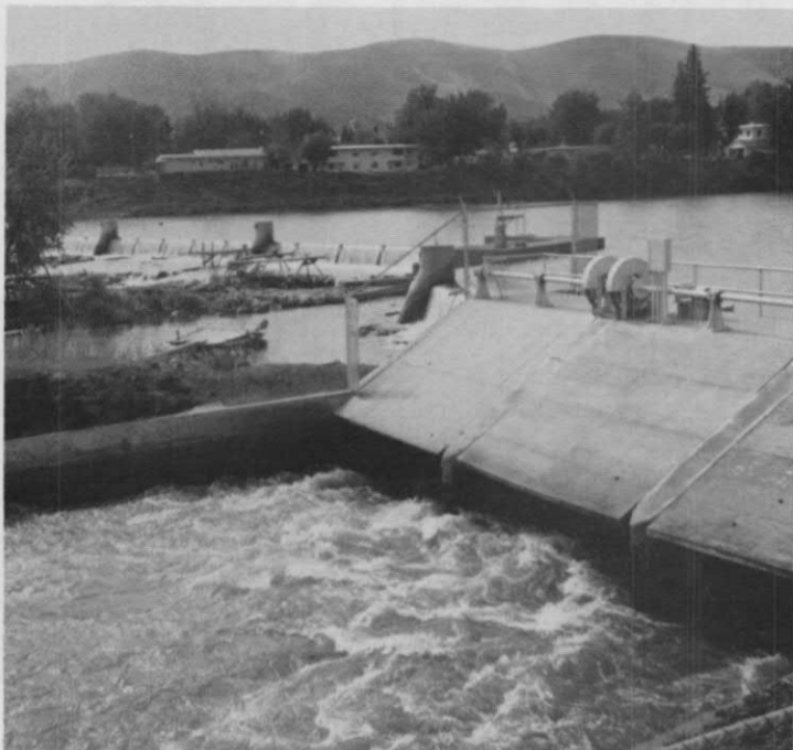
FIGURE 25.--Chandler Power Canal diversion from Yakima River at Prosser Diversion Dam.
