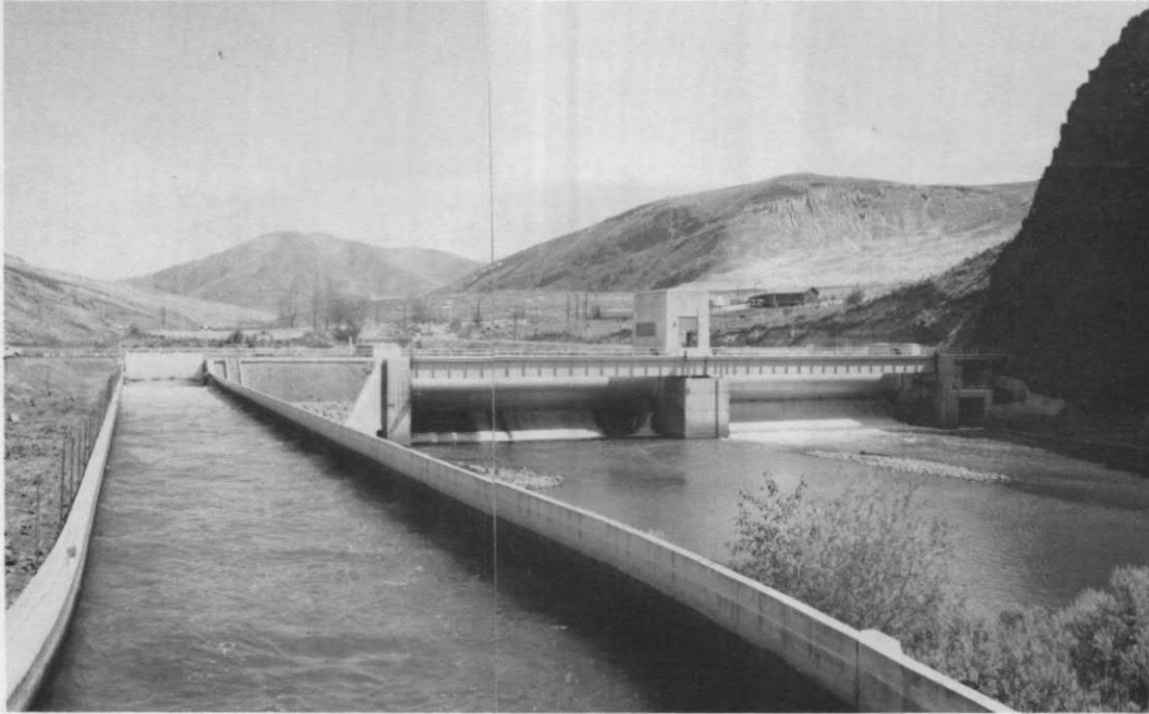
FIGURE 20.—Roza Canal diversion at Roza Dam on Yakima River.
