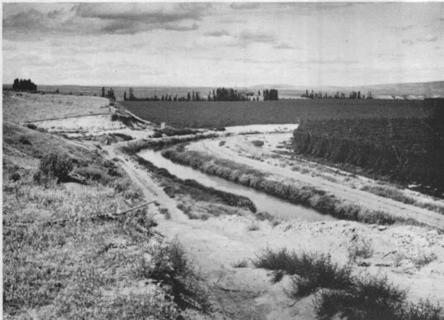
FIGURE 24.—Satus No. 2 Pump Canal.
