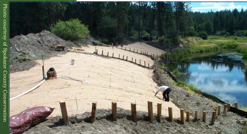
Erosion control fabric with barbs
