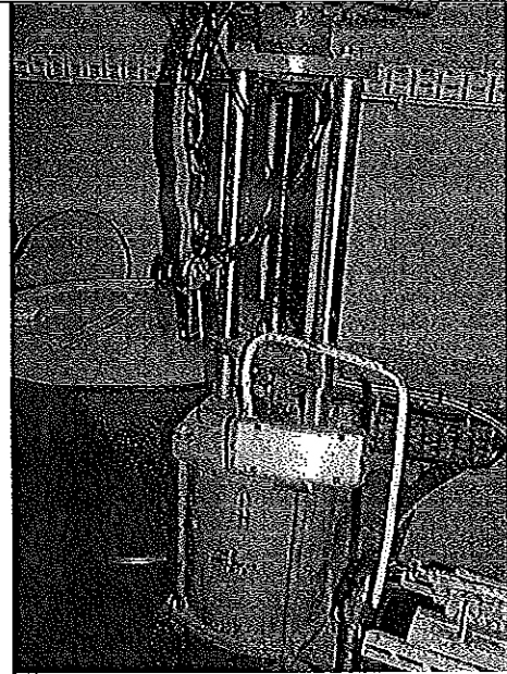
PHOTO #:12 DATE: SEPTEMBER 4, 2009 TAKEN BY: AMY JANKOWIAK FILE No.:P9040013 DESCRIPTION: DISCHARGE PORT WITH PADLOCK
