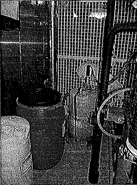
PHOTO #:29 DATE: JULY 19, 2009 TAKEN BY: AMY JANKOWIAK FILE No.:P7190053 DESCRIPTION: DRY CLEANING PERC WASTE COLLECTION
