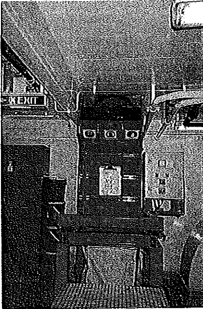
PHOTO #:13 DATE: AUGUST 08, 2009 TAKEN BY: AMY JANKOWIAK FILE No.:P8080013 DESCRIPTION: GLASS CRUSHER
