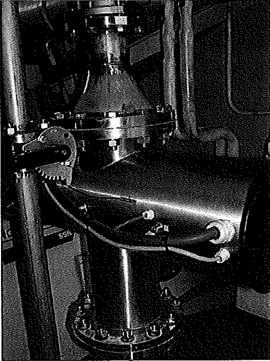
PHOTO #:17 DATE: AUGUST 16, 2010 TAKEN BY: AMY JANKOWIAK FILE No.: P8160020 DESCRIPTION: HAMWORTHY ULTRAVIOLET DISINFECTION UNIT
