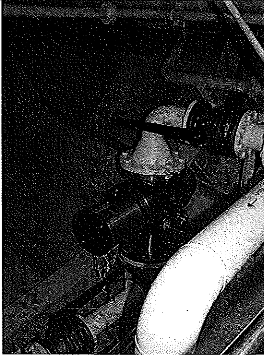
PHOTO #:21 DATE: SEPTEMBER 12, 2010 TAKEN BY: AMY JANKOWIAK FILE No.:P9120030 DESCRIPTION: ULTRAVIOLET LIGHT DISINFECTION UNIT
