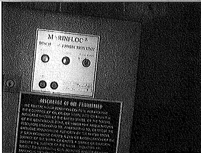
PHOTO #:15 DATE: JUNE 18, 2010 TAKEN BY: AMY JANKOWIAK FILE No.: P6180040 DESCRIPTION: OILY WATER SEPARATOR SYSTEM (OWS)
