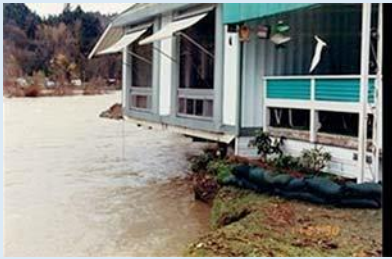
Cedar River flooding threatening mobile home park. The homes were purchased and removed, while the floodplain was reconnected.
