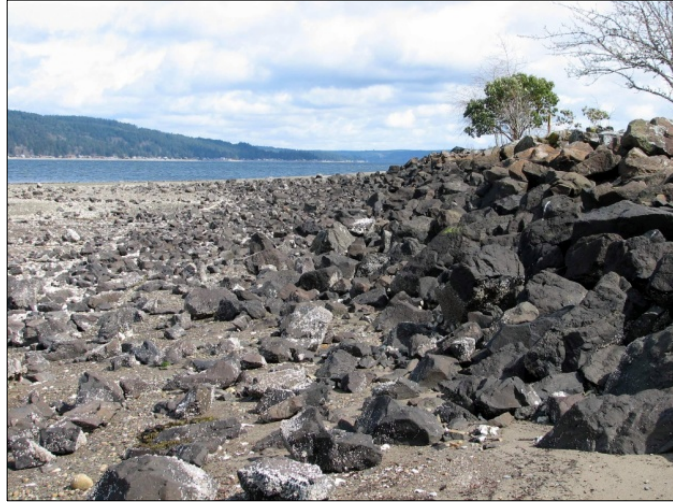
Figure 4: Replacing this riprap revetment at Twanoh State Park on Hood Canal could include shifting the structure landward, restoring the upper beach, replanting native vegetation, and removing loose riprap. (Hugh Shipman photo.)
