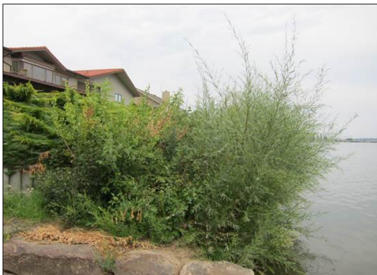
Figure 15-8: This soft shoreline stabilization stabilizes the bank of Moses Lake and helps to protect the house, a primary structure. Views from the house and the lawn above the retaining wall are not obstructed by the vegetation. The rocks in the foreground are at the property line. (Doug Pineo photo.)
