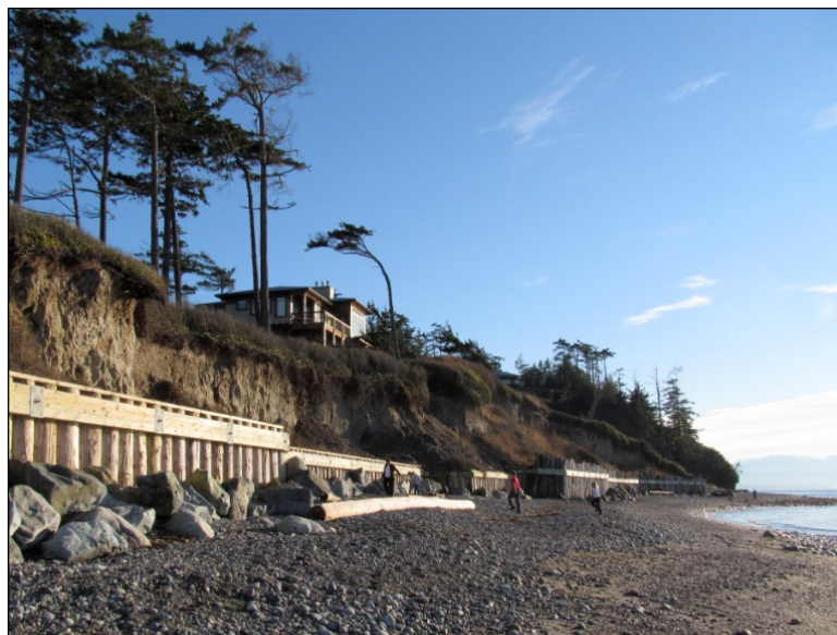
Figure 15-7: Although stabilization structures are often built and permitted on a site by site basis, on many shorelines this results in long stretches of armored shoreline. This example is from Whidbey Island; similar patterns can occur on lakes and rivers. (Hugh Shipman photo.)
