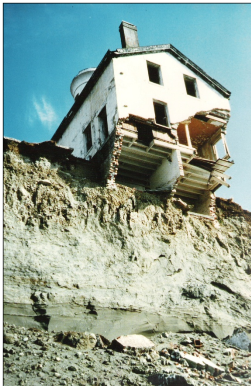
Figure 15-14: The old Smith Island lighthouse in the Strait of Juan de Fuca was clearly threatened by rapid erosion at the time of this photo in the 1980s and had already been replaced by a new structure farther landward. When structures are seriously threatened by erosion, relocation is often the best option. (Gerald Thorsen photo).
