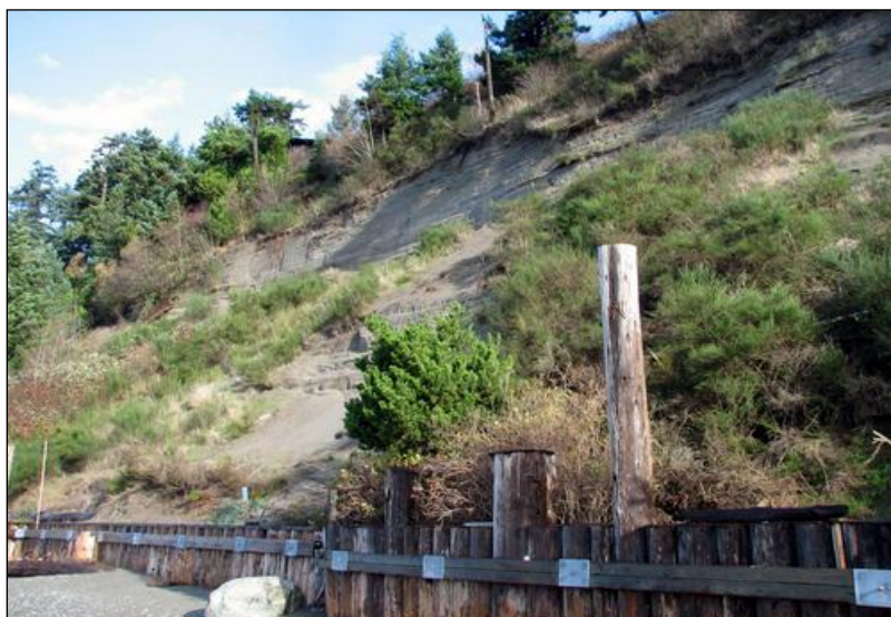
Figure 15-4: The timber pile bulkhead prevents material from a feeder bluff from reaching the littoral system. Erosion is an important geological process that forms and maintains shoreline ecosystems. (Hugh Shipman photo.)
