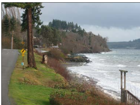
Figure 15-12: This county road follows the top edge of a bluff on Hood Canal. Erosion impacts the road in some locations. Stabilization may be justified because of the public benefit conferred by the road. However, protecting a road in this location in the long-term will be extremely costly and will adversely impact the shoreline. Realignment of the road, perhaps combined with softer methods of erosion control, may be a more judicious response.
