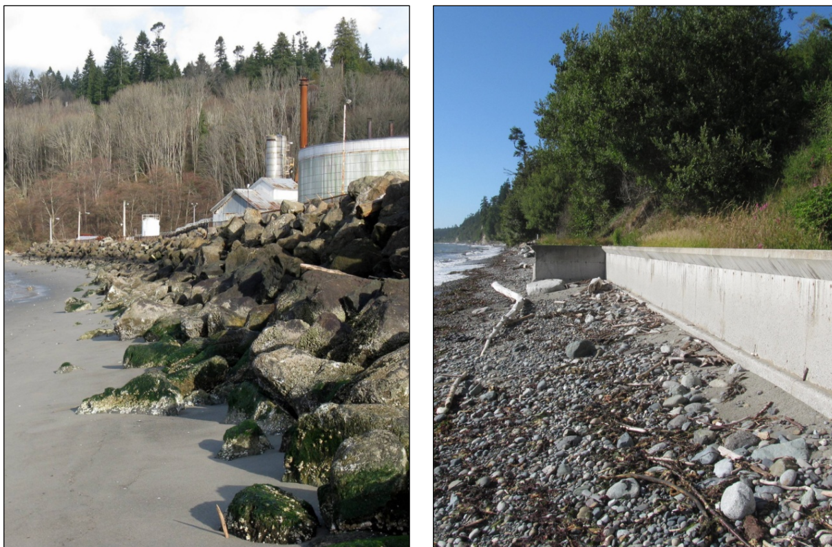
Figure 15-2: Riprap revetment protects the petroleum processing facility at Point Wells, Snohomish County (left). A residential bulkhead sits at the toe of a bluff on Whidbey Island (right). (Hugh Shipman photos.)
