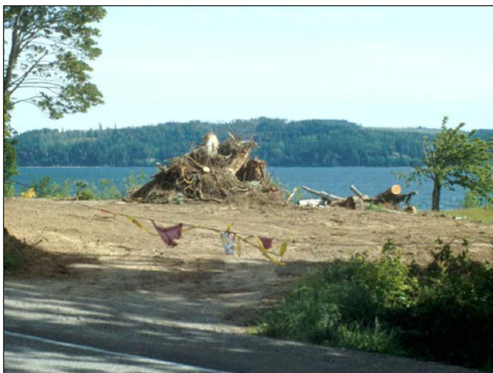
Figure 15-18: Removal of vegetation, disturbance of soils, and altered upland runoff can all contribute to shoreline erosion. These types of problems should be addressed before resorting to a stabilization structure such as a bulkhead or revetment. (Hugh Shipman photo.)
