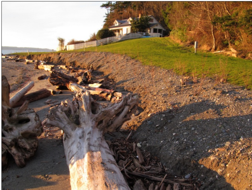
Figure 1: This shoreline on southern Whidbey Island was previously protected with a timber bulkhead. Rather than replace it, the owner reconfigured the bank, planted vegetation, and accepted that a modest level of erosion would continue without jeopardizing upland improvements. (Hugh Shipman photo.)
