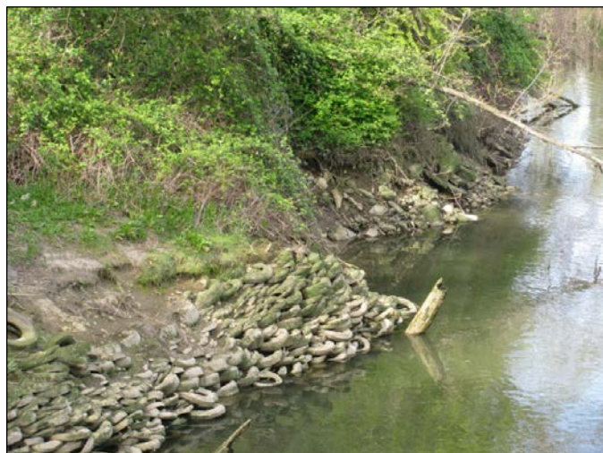
Figure 15-6: Bank stabilization along the Duwamish River uses debris and old tires. This type of bank stabilization has adverse environmental and aesthetic impacts. (Hugh Shipman photo.)
