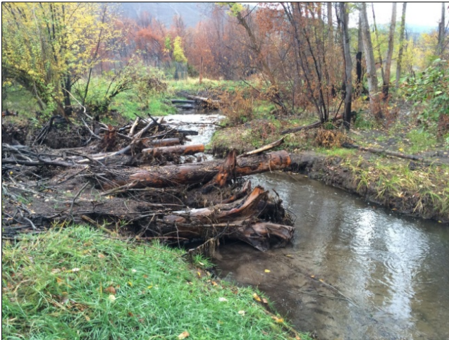
Figure 4: Erosion control structure was constructed by anchoring large wood along Beaver Creek in the Methow Valley. (Hugh Shipman photo.)
