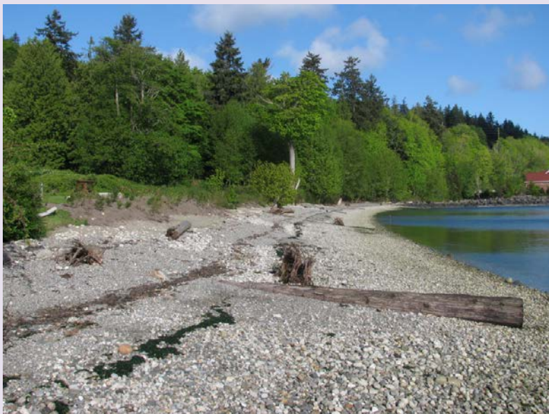
Shoreline stabilization at this site in Anacortes employs plantings, added beach gravel, and strategically located large wood. (Hugh Shipman photo.)
