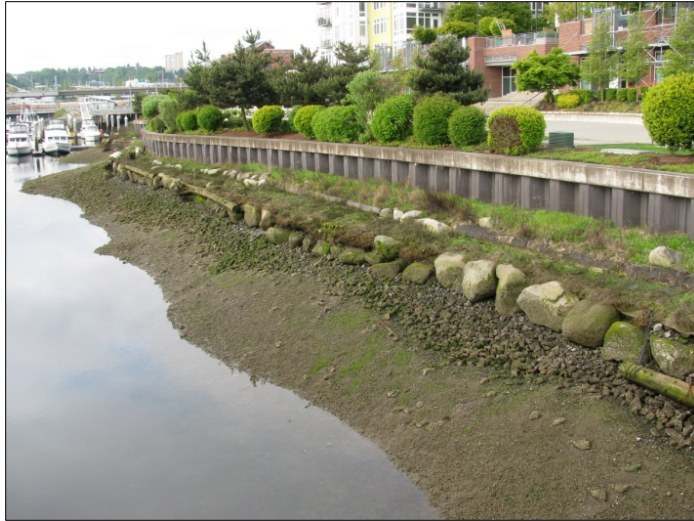
Figure 2: A number of techniques have been used on this Tacoma shoreline to provide ecological functions, while also managing erosion on a heavily developed waterfront. The bulkhead has been kept landward and wood and marsh vegetation have been installed along the water. (Hugh Shipman photo.)
