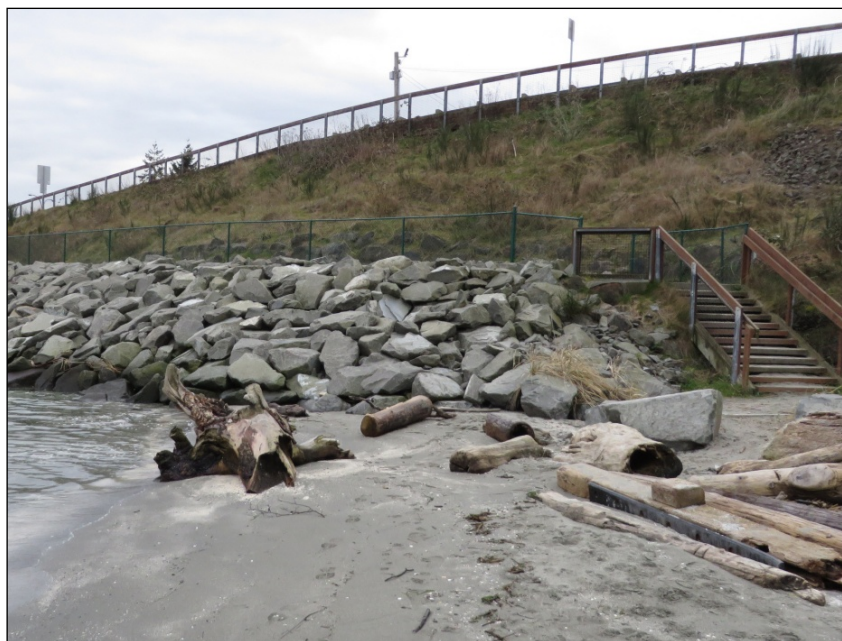
Figure 15-20: Public access to the adjacent beach was built into this stabilized slope at the Kingston ferry terminal. (Hugh Shipman photo.)
