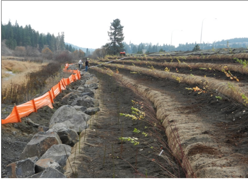
Figure 3: Bank stabilization along Hangman Creek in Spokane County includes soil lifts, a rock toe and plants. The project, which was completed in 2014, will reduce erosion and stabilize the stream bank adjacent to U.S. 195. (Mike Maher photo.)
