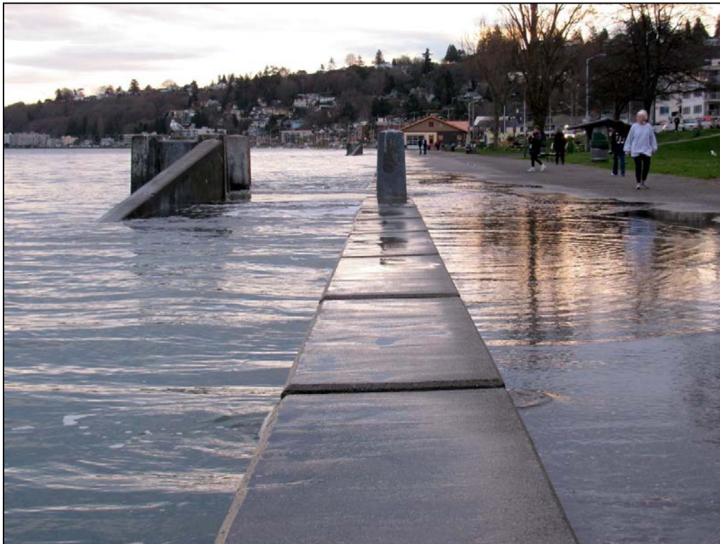
Figure A – 1: An unusually high tide in January 2010 caused water to spill over the seawall at Alki Beach in Seattle. Even modestly higher sea levels will cause the frequency of events such as this to increase, along with the potential for associated damage. (Photo by Hugh Shipman.)
