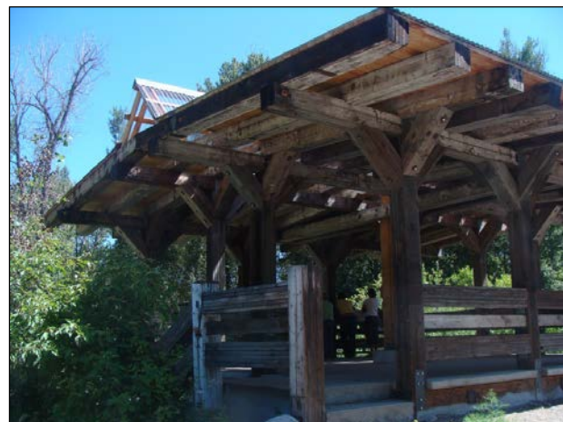
Figure 9-9: Viewing towers can provide visual public access at critical areas, industrial areas, and locations like this one on the Twisp River. (Photo by Department of Ecology.)
