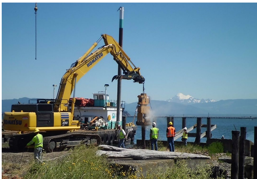
Figure 16-4. Piling removal using the vibratory hammer method.
