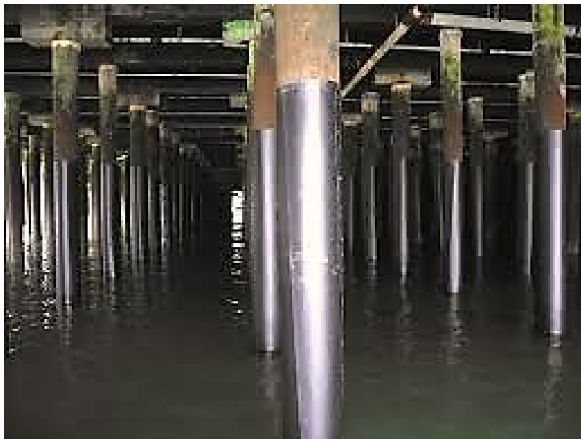
Figure 16-2. Wrapped piling at the Squamish Terminal in Squamish, British Columbia.
