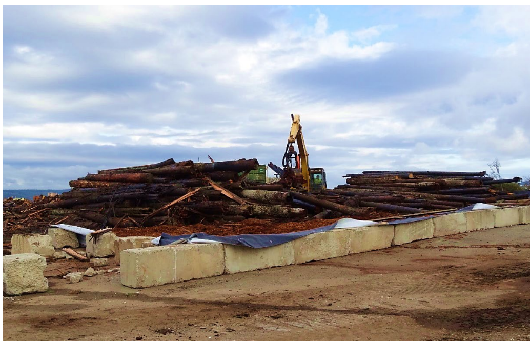
Figure 16-9. Piling removal containment area at the former mill site in Port Gamble Bay, WA. The containment area is constructed of ecology blocks, a synthetic liner, and wood mulch that prevent the release of sawdust, debris, splintered wood, and unfiltered water.
