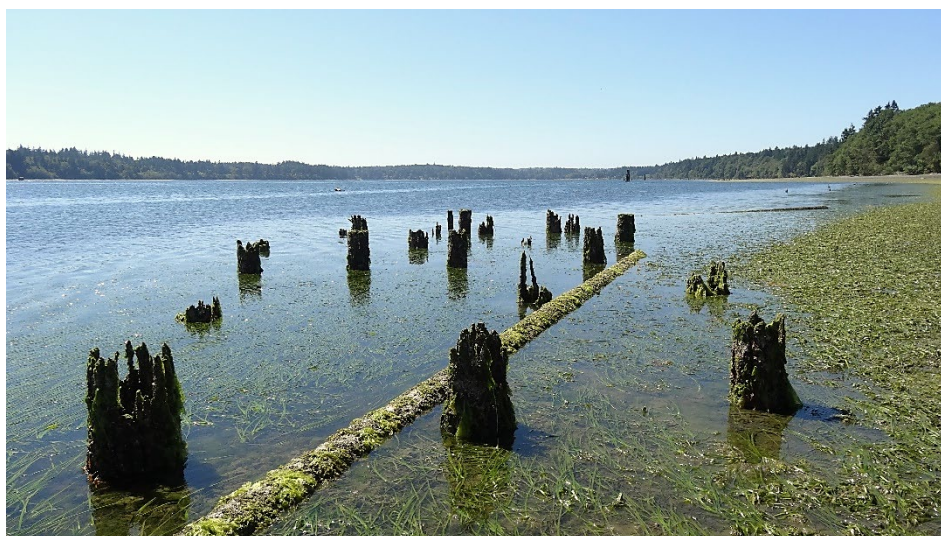
Figure 16-6. Decayed piling stubs in eelgrass at the former Port Gamble sawmill in Port Gamble, WA.
