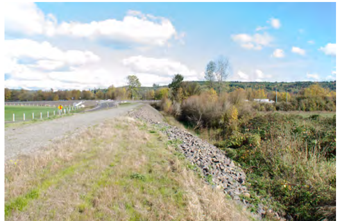
View looking north from atop the Chehalis-Centralia Airport Levee
