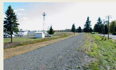
Chehalis-Centralia Airport Levee
