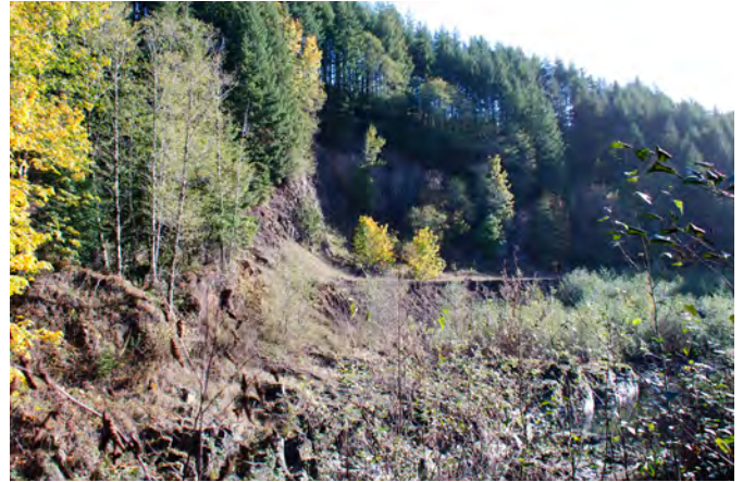
View looking east, within the outer footprint of potential flood retention facility
