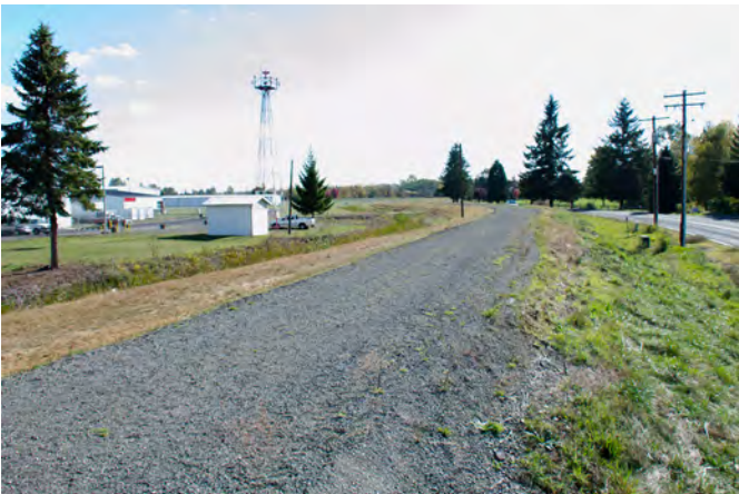
View looking south from atop the Chehalis-Centralia Airport Levee
