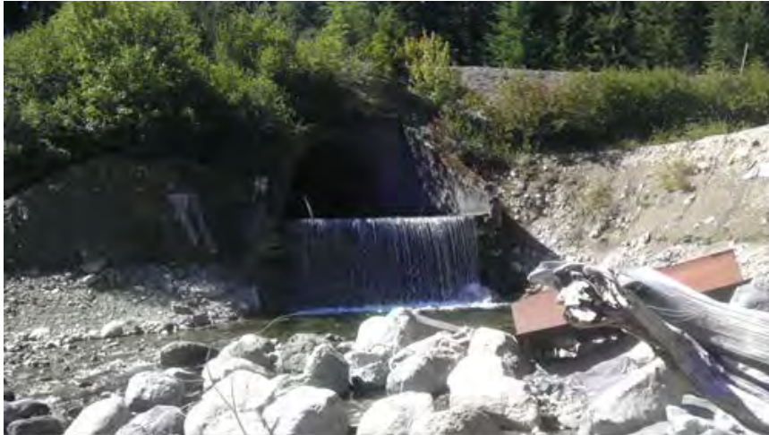
Figure 3-10. Existing passage barrier at Cold Creek culvert.
