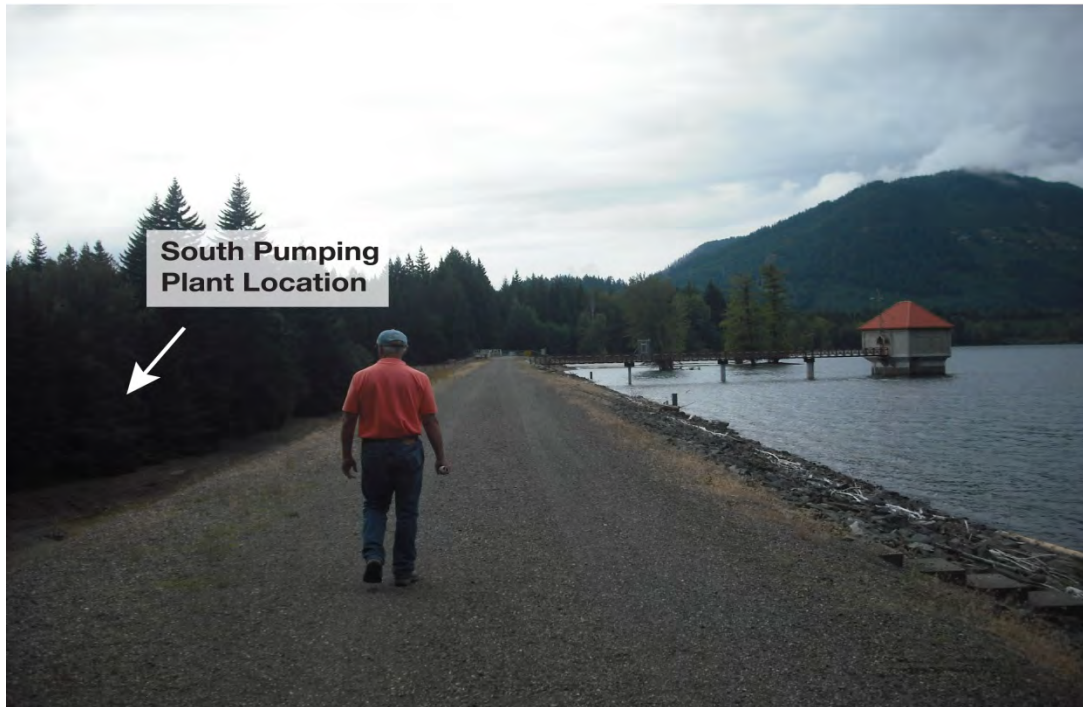
Figure 4-18. South Pumping Plant Location (South of Kachess Dam)
