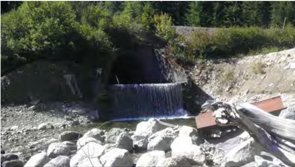
Figure 3-36. View of Palouse to Cascades State Park Trail and Cold Creek Culvert
