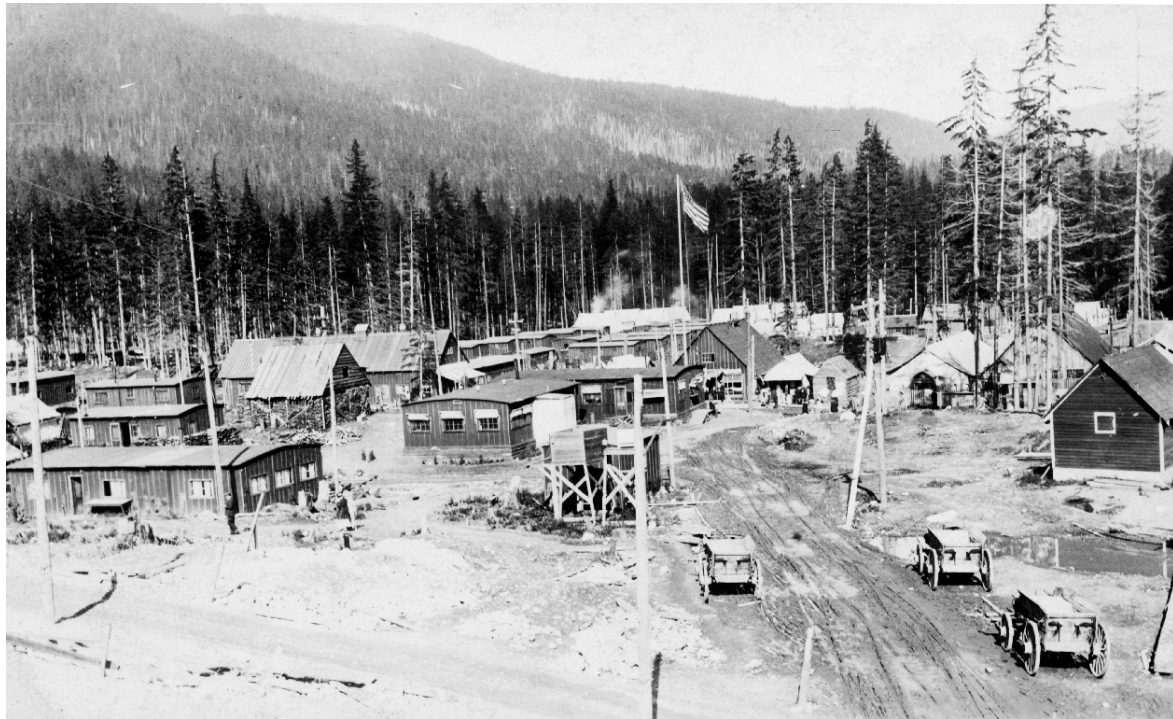
Figure 3-50. View of Keechelus Construction Camp circa 1914
