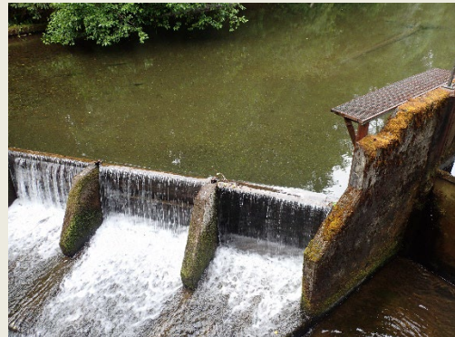
This structure on Bingham Creek has a fish ladder and smolt trap that have provided approximately 40 years of wild coho salmon life-cycle monitoring information.
