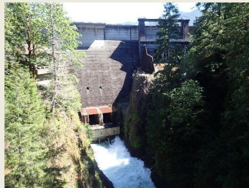
Wynoochee Dam is a fish passage barrier and affects gravel and wood loading downstream.
