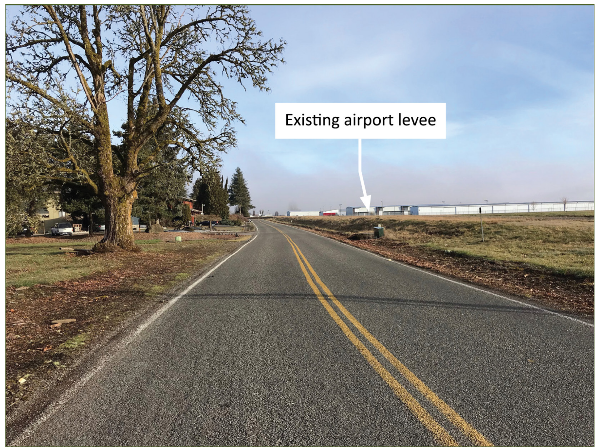
View of Airport Levee from NW Airport Road Looking North
