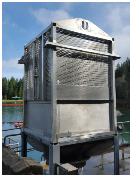
Figure 4-22 Example Fish Hopper at Cushman Adult Collection Facility (Courtesy of Tacoma Power)
