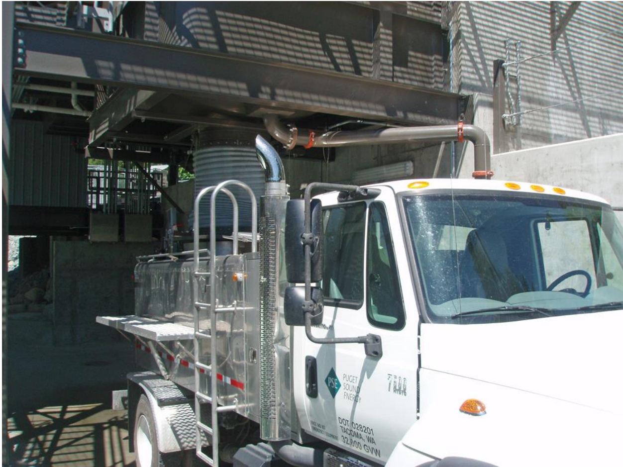
Figure 4-14 Water-to-Water Transfer from Holding Tank to Transport Truck, Courtesy of Puget Sound Energy
