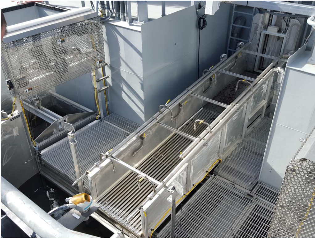
Figure 4-21 Example Grading Flume and Holding Pools Present on the Cushman FSC
