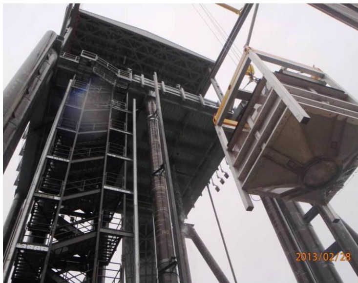
Figure 4-23 Example process of Lifting Hopper to Transport Vehicle at Swift FSC (Courtesy of PacifiCorp)
