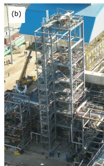
Fig. 1. Methanol plant overview for Flowsheets 1–3 : (a) diagram of the unit operations for Flowsheets 1–3 ; (b) picture of a SMR + ATR used in Flowsheet 3
