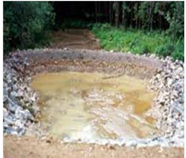
Photo 5. A below-field SCoB in a drainageway.
