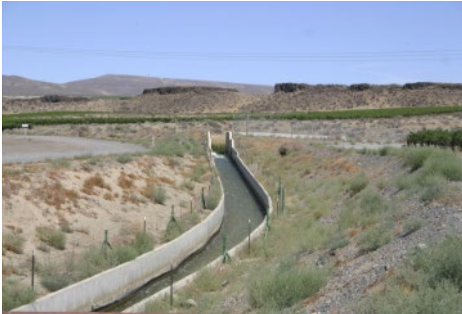
Figure 9. Example of a lined waterway (USDA NRCS 2020).
