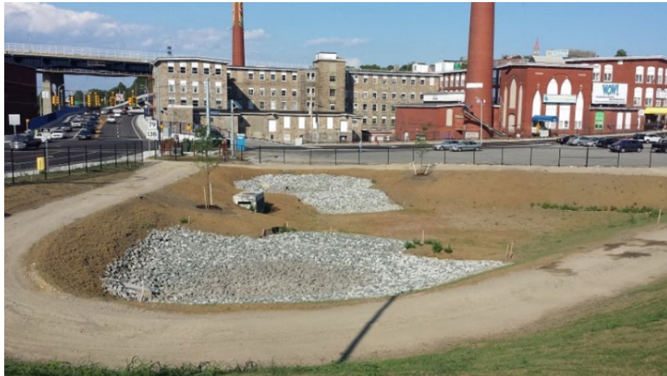
Figure 16. Infiltration Basins are more common in urban setting as shown here but can be applied to agricultural settings as well where they can effectively draw water into the ground with vegetation and gravel. The image shows the flattened gravel before being covered with soil and vegetation (EPA, Credit Massachusetts Dep. of Transportation)
