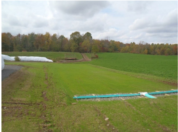
Figure 17: VTAs require larger areas of flat land covered in vegetation to infiltrate water. Diversion methods such as underground outlets can outlet water (Wayne County Soil & Water Conservation District).
