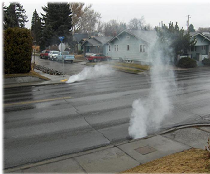
Figure 35: Illicit connection smoke testing.
