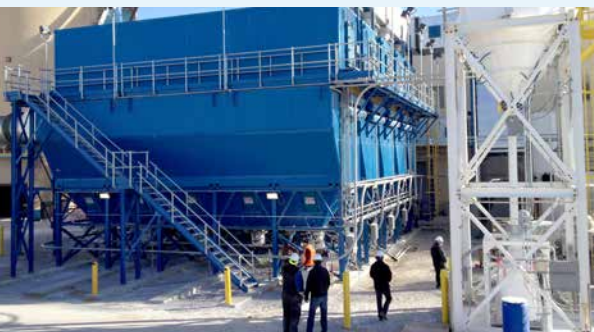
Reverse pulse-jet cleaning mechanism for the filter tubes. Filter tube wall is 3/4" thick with catalyst embedded inside.
