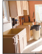
OKANOGAN A kitchen remodel is in progress, but insulation is
