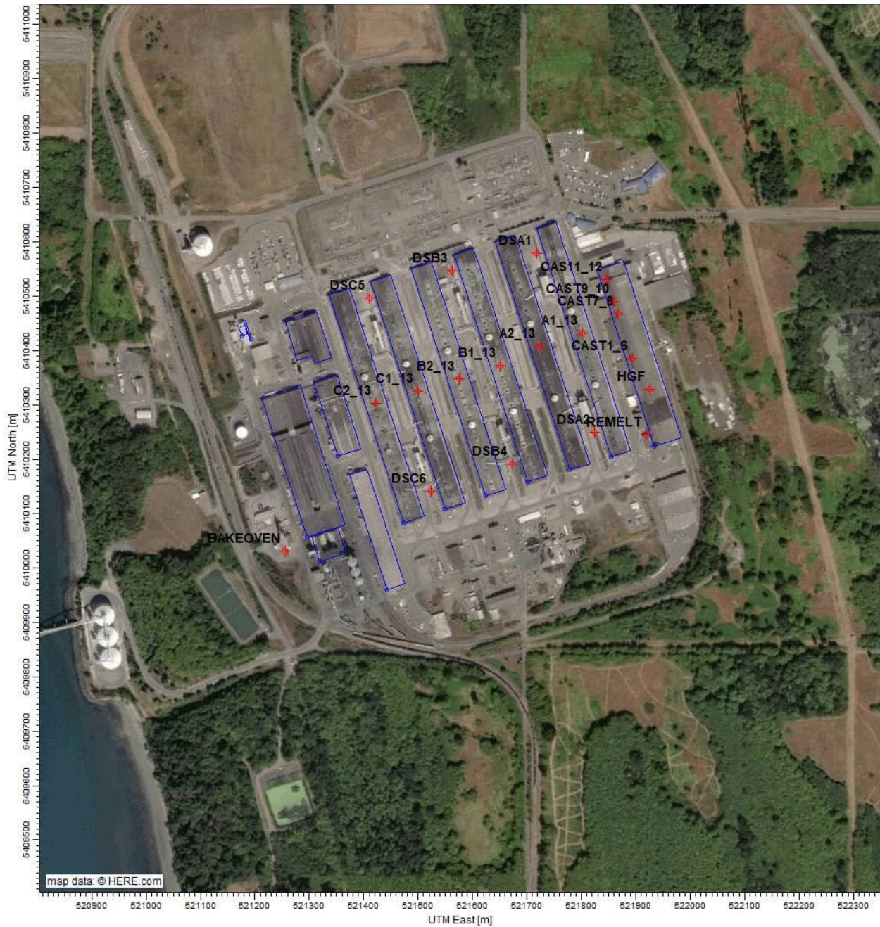
Figure 2-2: Aerial View of Intalco Buildings and SO 2 Emission Sources for Modeling
