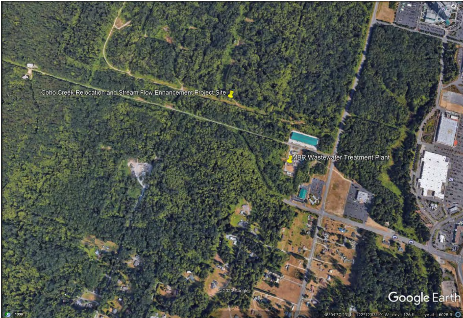
Figure 3. Coho Creek Relocation and Streamflow Enhancement Project Site
