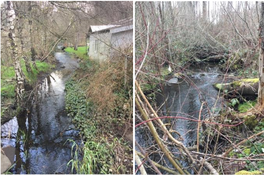
Photograph 4 (left). Riparian intrusion from residential structure just upstream from Site 2 (photograph taken March 25, 2020).
