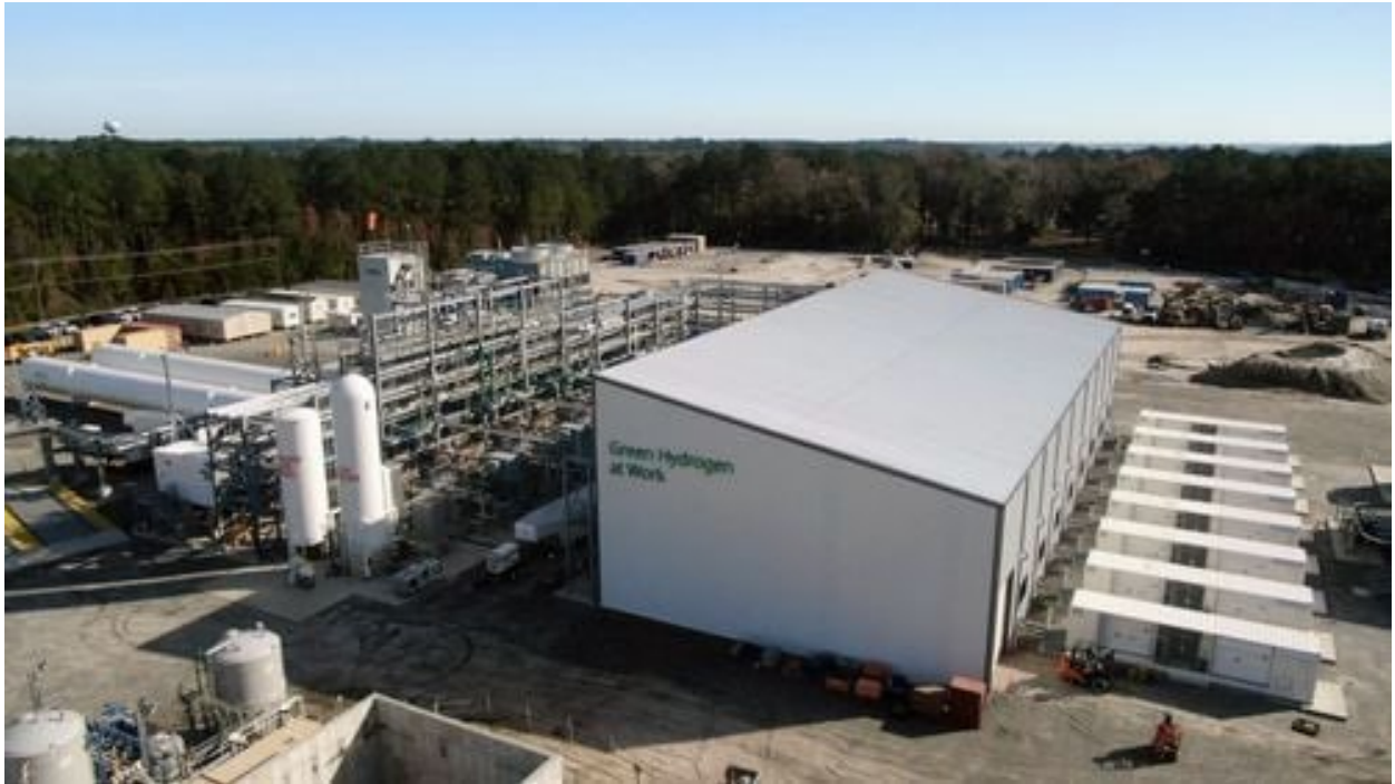
Figure 6. Electrolysis facility – Plug Power – Woodbine, GA
