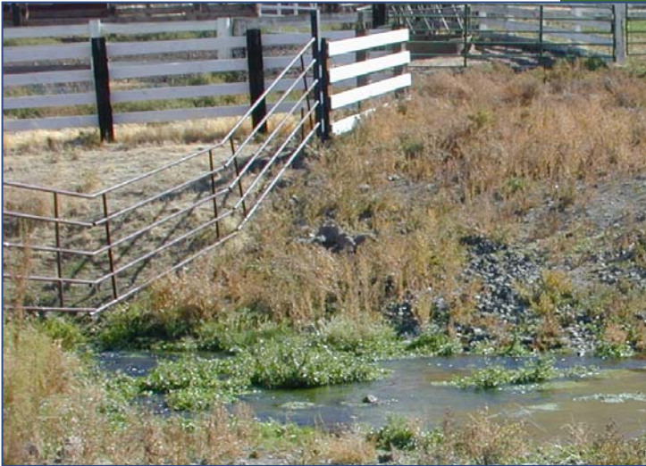
Tube gates hung from cable next to hardened crossing
