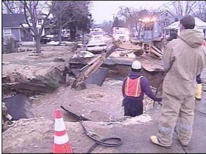
Figure 2: Water line break repair
