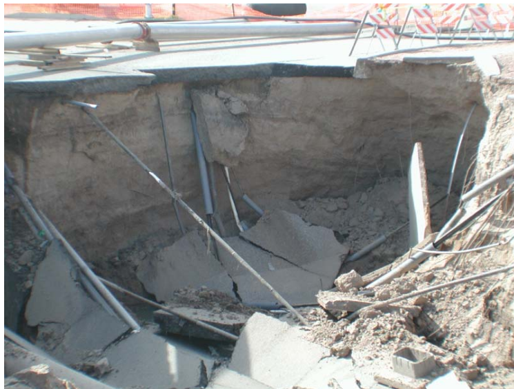
Figure 6: Collateral utility damage due to sewer collapse
