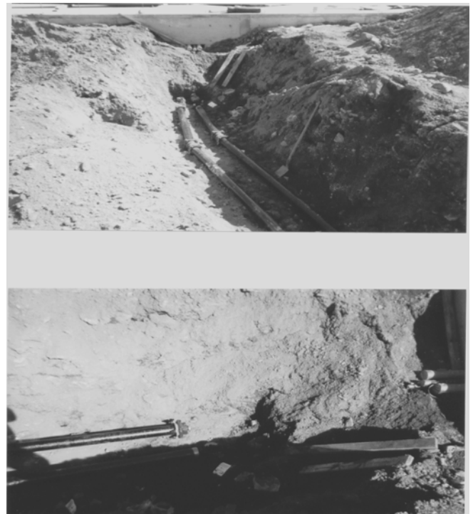
Figure 26: Field conditions - typical trench surcharge
