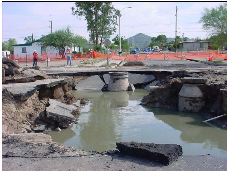
Figure 3: Sewer break
