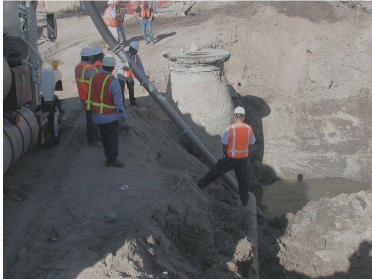
Figure 5: Waterline exposed by sewer collapse
