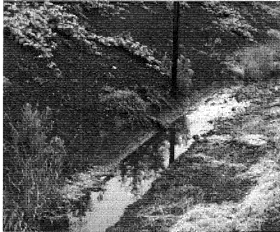
Photo #3: Highway 213/Clackamas Community College (CCC) Site. Photo shows mulch shedding off the embankment into the drainage ditch. Water can be seen flowing in the bottom of the ditch to a storm sewer.
