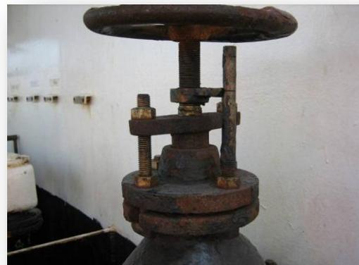
*Figure 4. No. 4 starboard main deck fuel oil tank valve. Note the indicator (valve position indicator) mounted on the shaft of the valve stem.*
