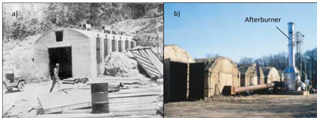
**Figure 44.** Concrete kiln (Missouri type) a) 100 cord capacity kiln without afterburner (Toole et al., 1961) and b) with afterburner (Source: <http://www.dnr.mo.gov/env/apcp/1999%20AnnualReport/99AirQualityHiLites.pdf>, date accessed February 6, 2011).
