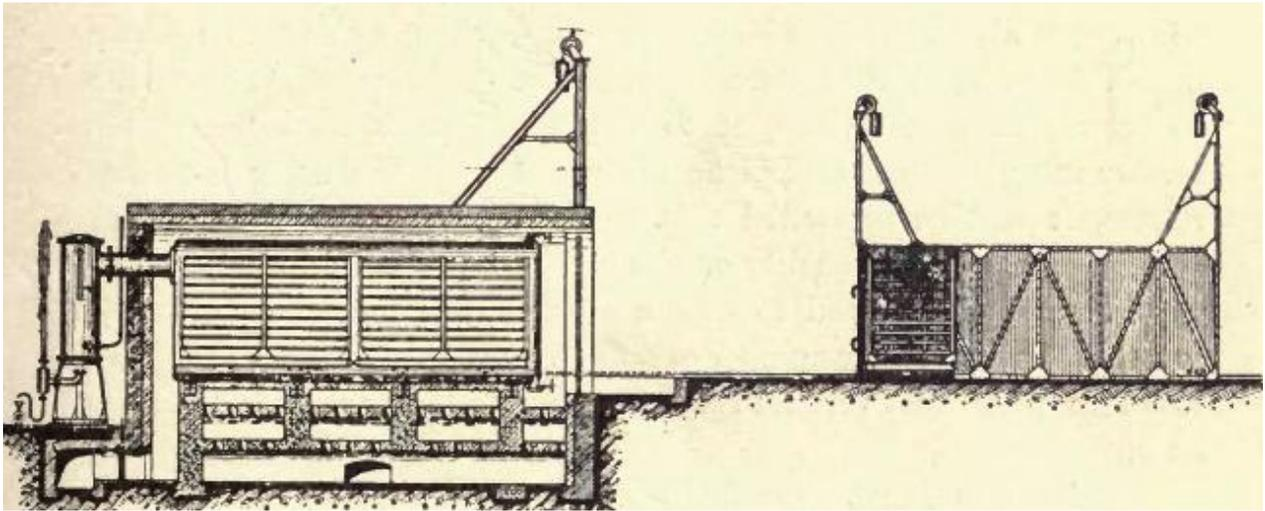
**Figure 71.** Retort for carbonization of small wood waste, and coolers for cooling the retorts after an operation (Dumesny and Noyer, 1908).
