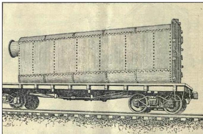
**Figure 21.** A semi-portable retort (Veitch, 1907)
