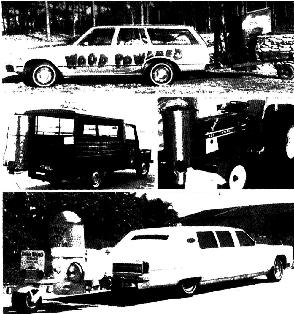
**Figure 80.** Vehicle gasifiers constructed after the fuel crisis in the 1970s. (SERI, 1988).
