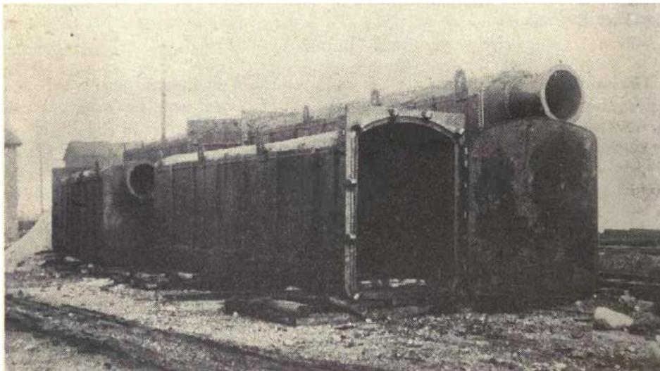
**Figure 50.** Ovens of a six-cord capacity retort awaiting installation (Bates, 1922).
