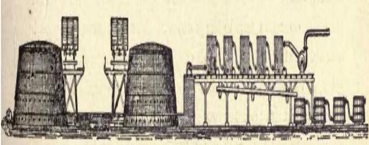
**Figure 45.** Masonry stack ovens (American “beehive” kilns) or furnaces for wood distillation on very large scale and appropriate condensation plant (Dumesny and Noyer, 1908).
