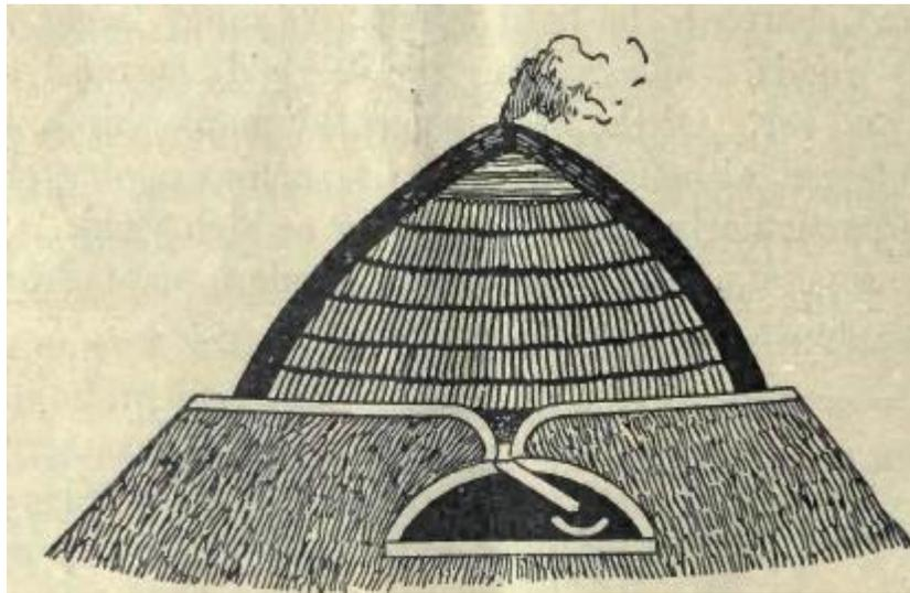
**Figure 34.** Early form of kiln in which biochar and tar are recovered (Veitch, 1907).
