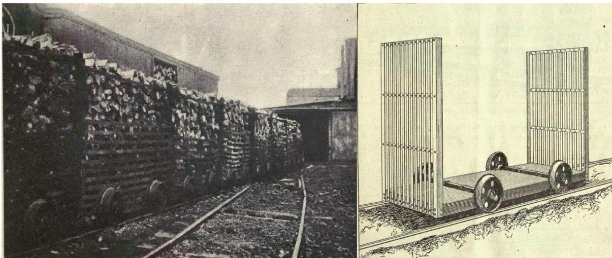
**Figure 29.** Cars used to load wood into the oven (Bates 1922, Veitch 1907).
