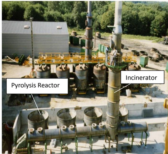
**Figure 7.** A CML Process under construction (CIRAD and Innov-energies, 2007).
