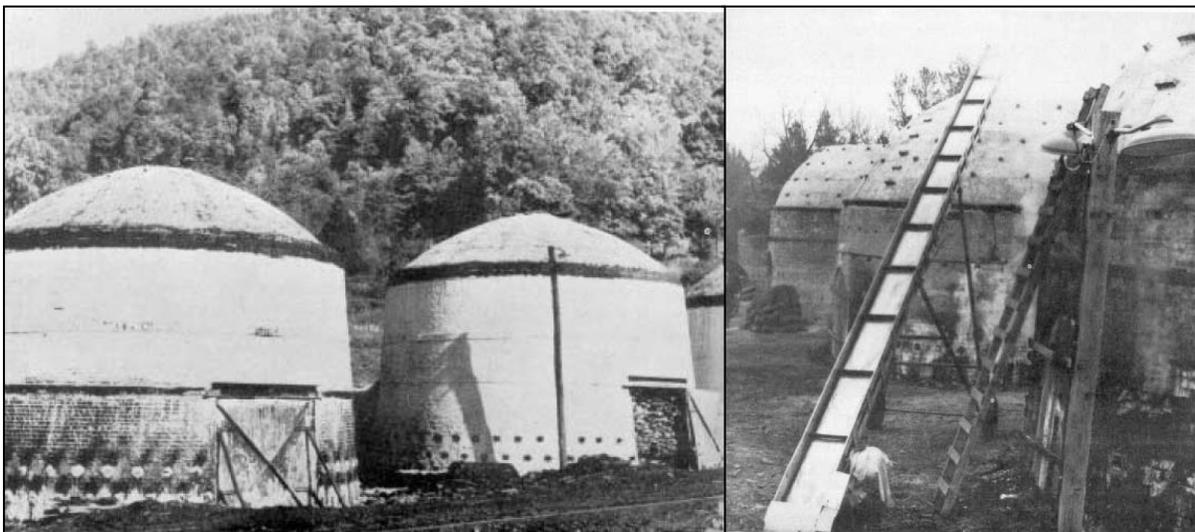
**Figure 46.** Stationary large “American” kilns for biochar production (Klark, 1925).
