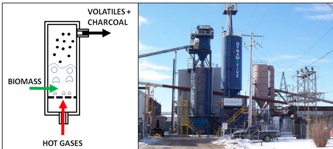
**Figure 74.** Fluidized bed reactors (Dynamotive, <http://www.dynamotive.com/technology/>, date accessed: Nov. 13, 2010).
