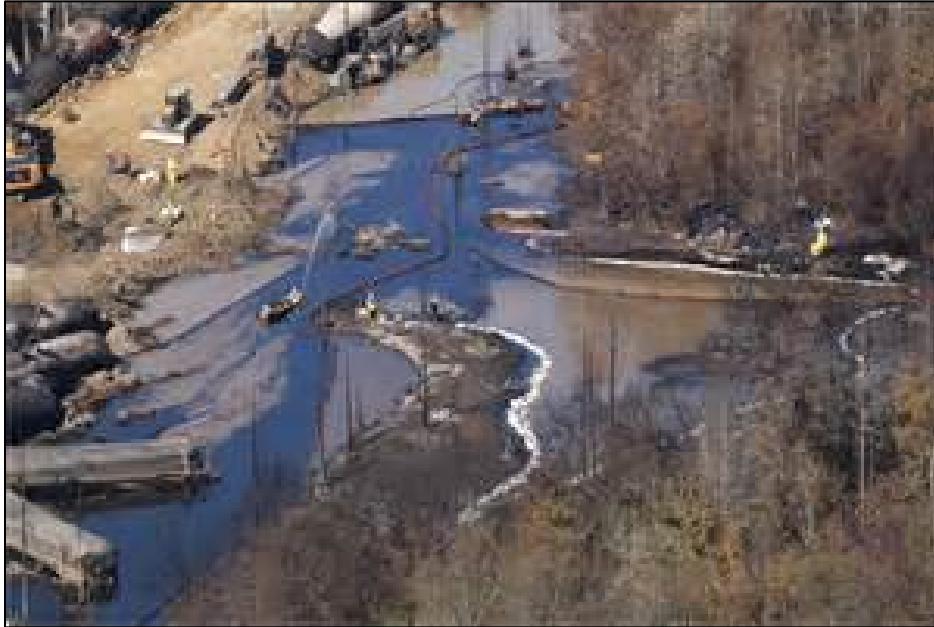
Figure 144: Aliceville, Alabama, Bakken Spill Cleanup: Booming, Vacuum Trucks, Water Spraying 535
